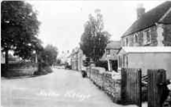
The Chestnuts-coping stones missing
